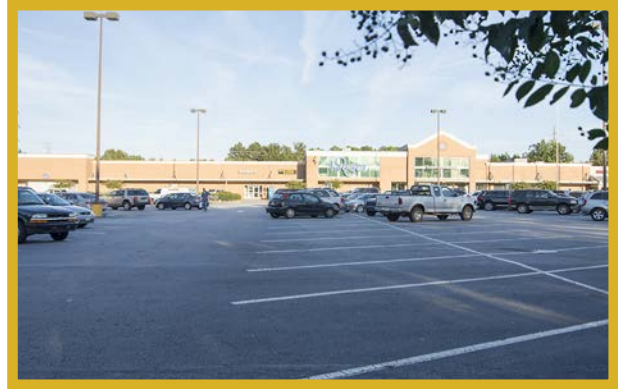
Kruger Anchored Center Directly Across Street from Subject Property
